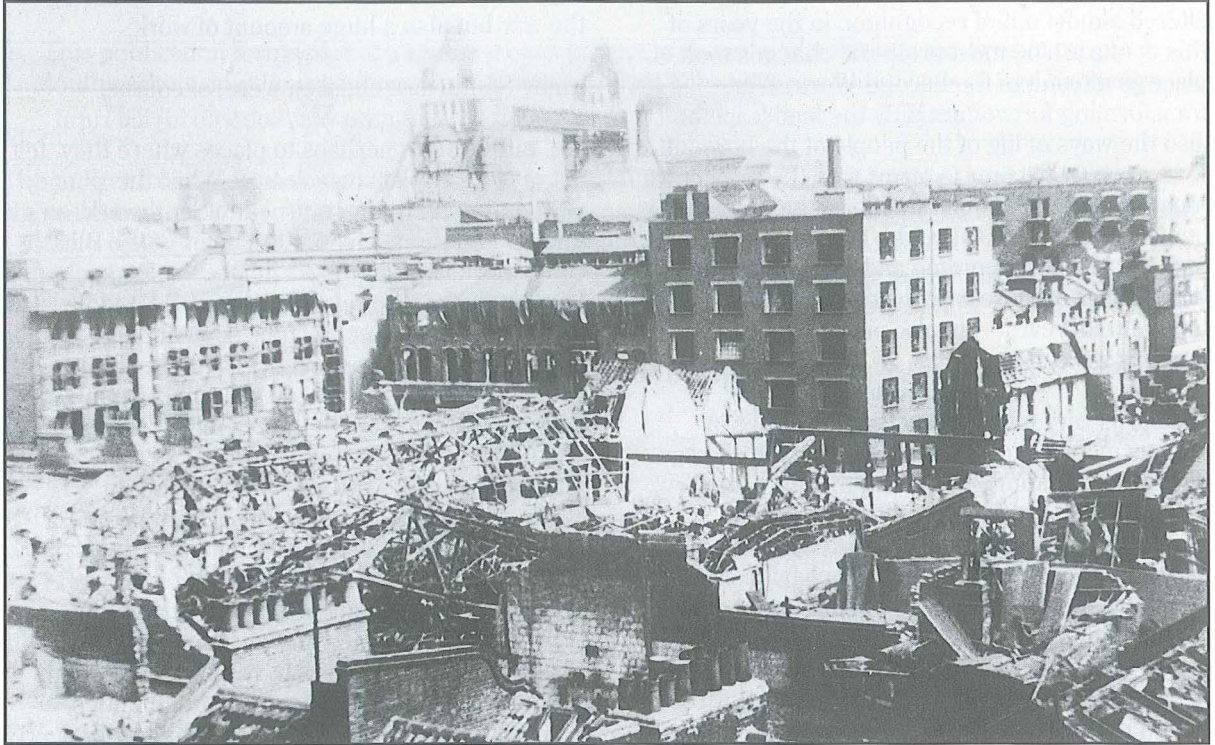
A view looking north towards Tower Bridge across the Gainsford Street area of Bermondsey.
