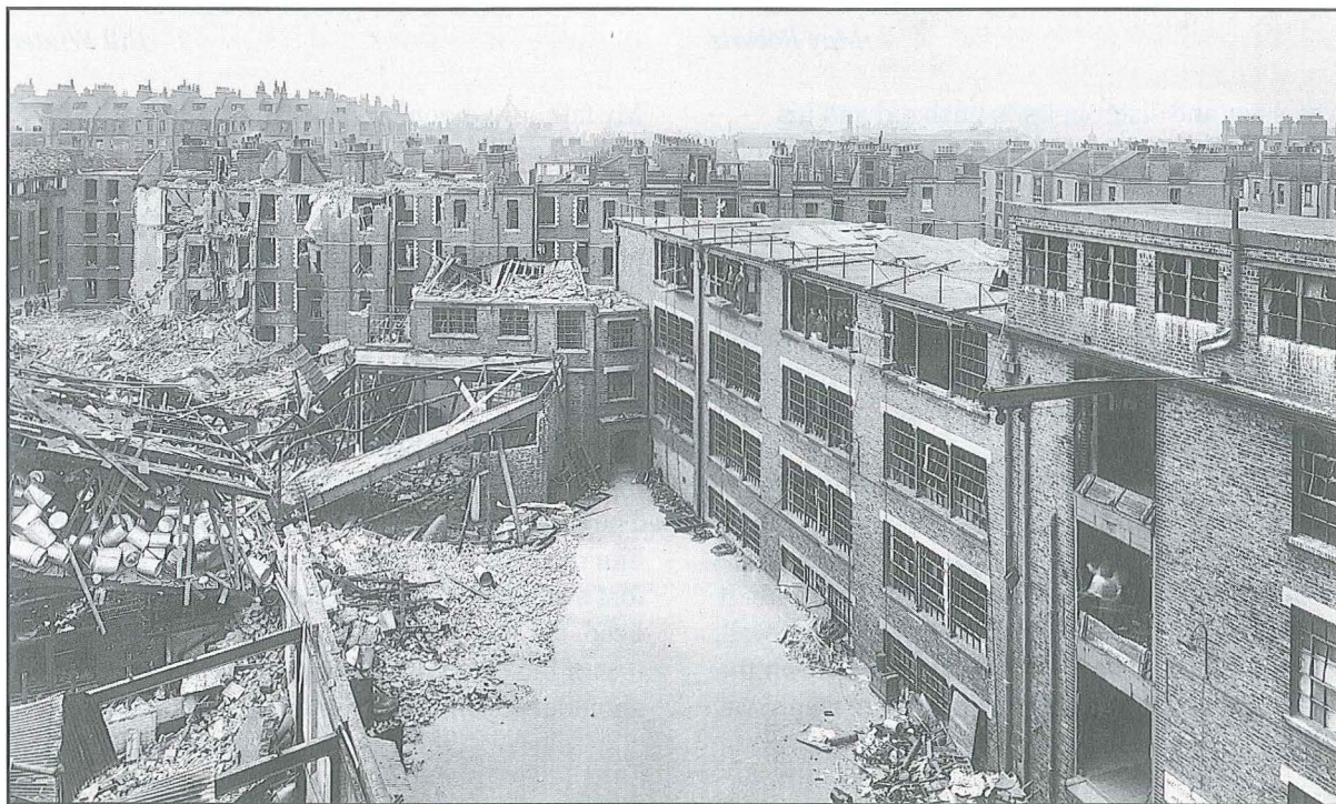
The devastation of Barrow, Hepburn and Gales leather manufacturers, in Grange Road, May 1941.
