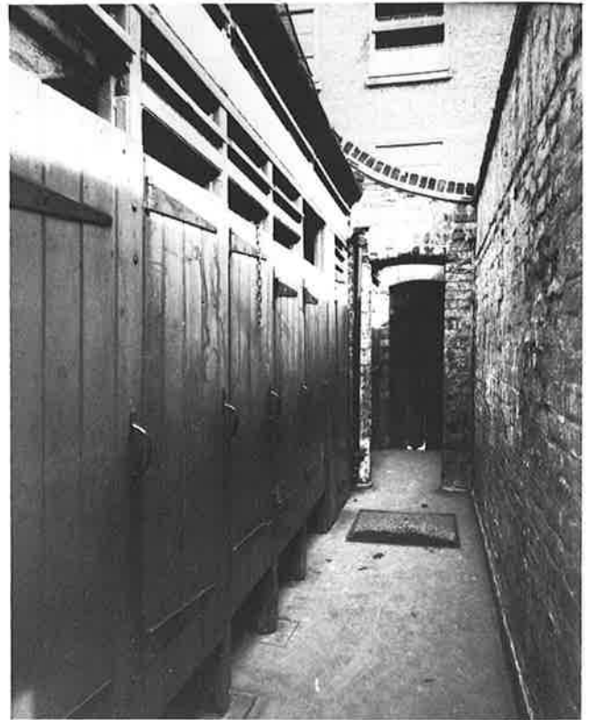
Belleville School. Water Closets. 1936.
